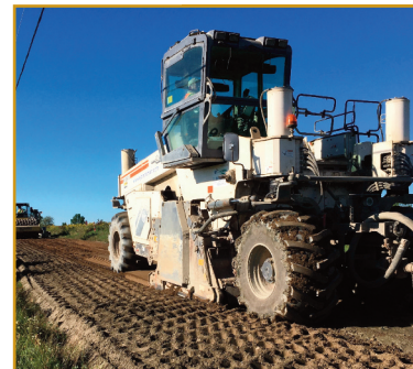
Step 3: Grind the Slurry into the Prepared Road Base
