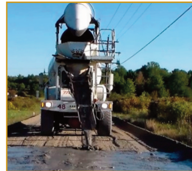
Step 2: Apply Cement Slurry to Prepared Road Base
