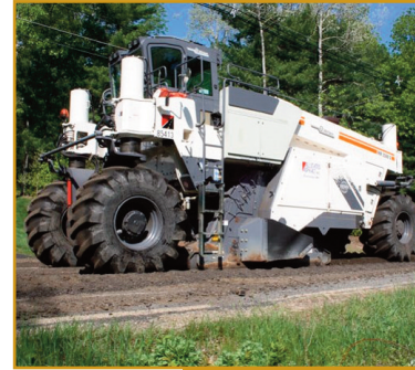
Step 1: Grind the Existing Pavement
