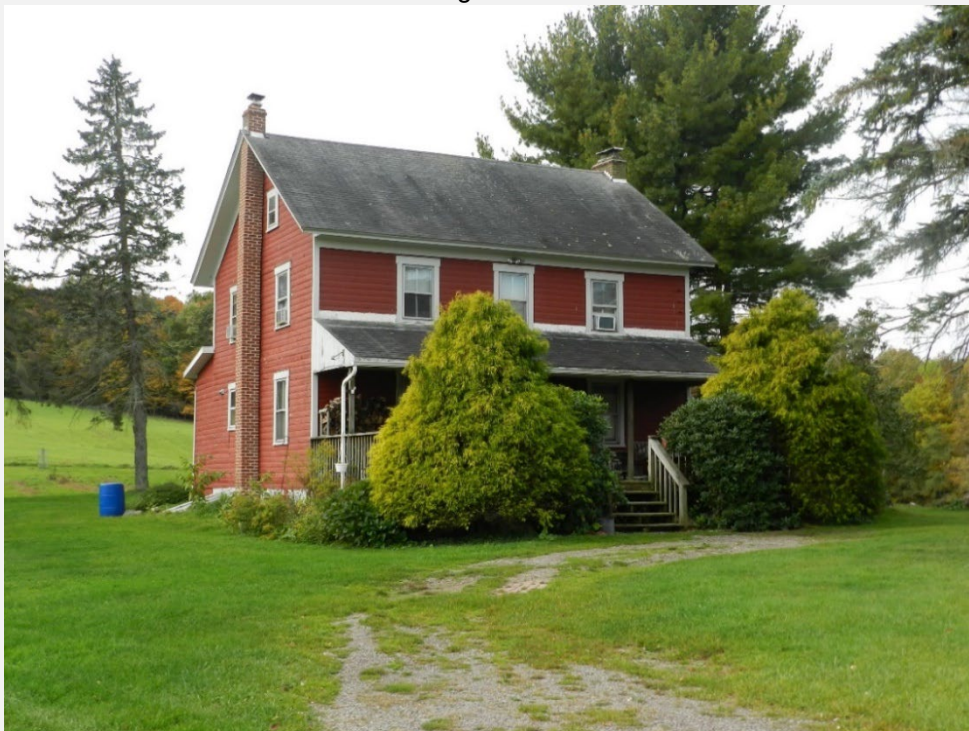
Photo 2. The dwelling on the Sidney Markowitz Farm/Newman Farm (G-I-A-139), looking southwest.
