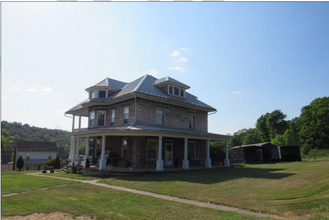
Photograph 2. South (front) and east elevations of the farmhouse, facing northwest.
