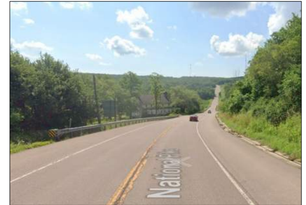
The National Road National Pike / Alt 40, MD NRHP eligible
