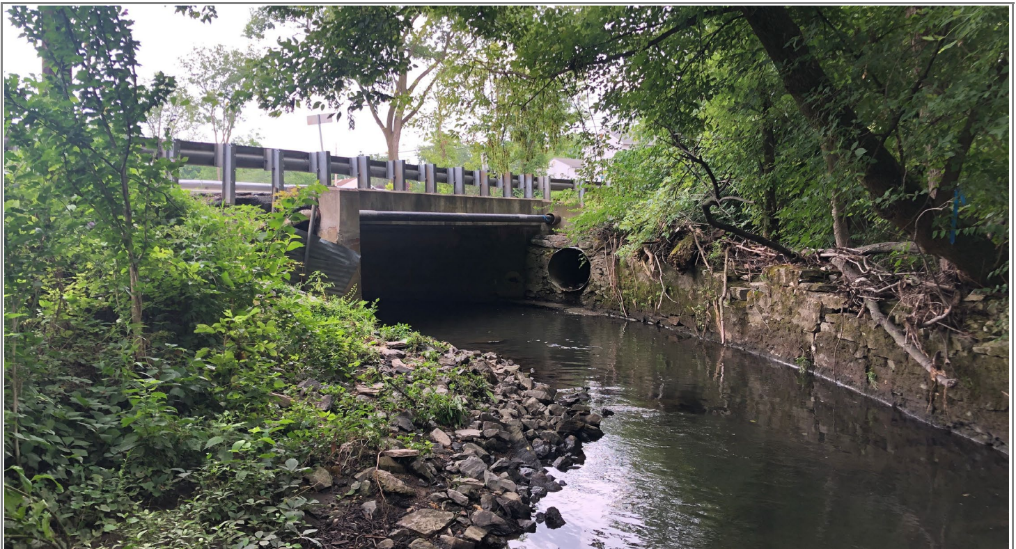
Photo 4 : View of Existing Bridge Over Quittapahilla Creek (Downstream Side)
