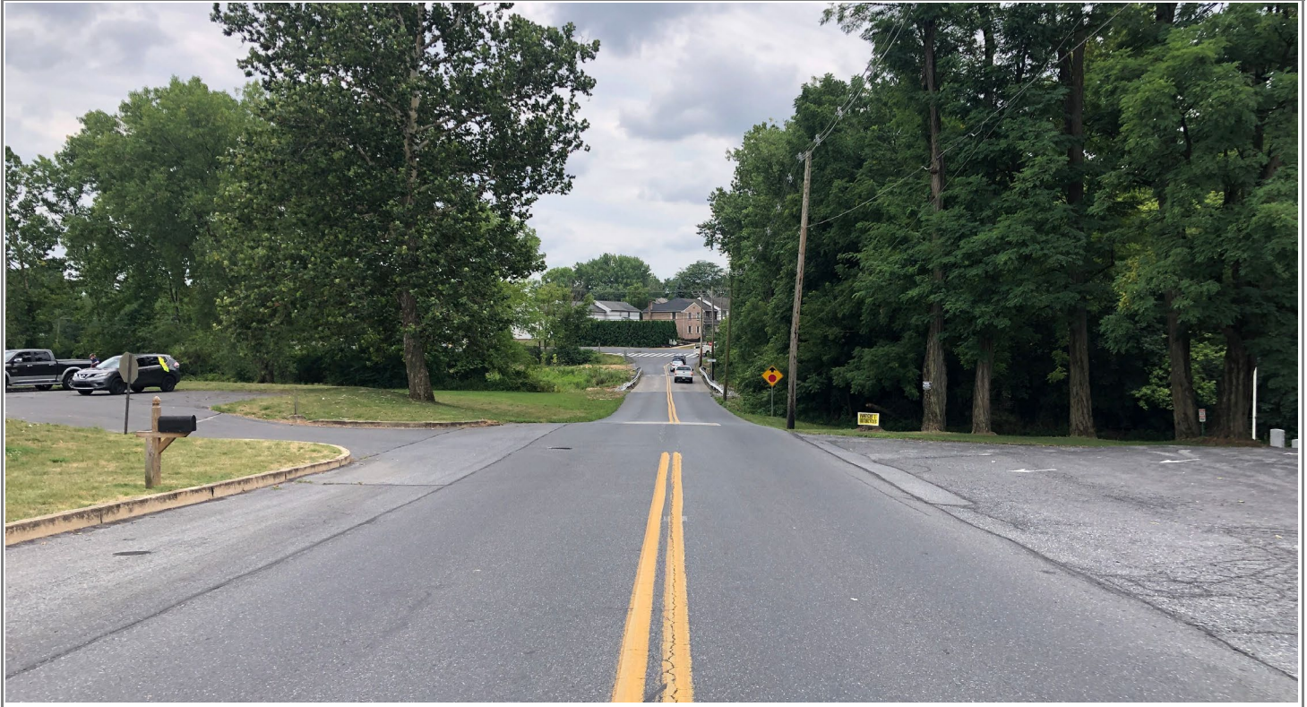
Photo 1 : View of 22nd Street Towards Chestnut Street
