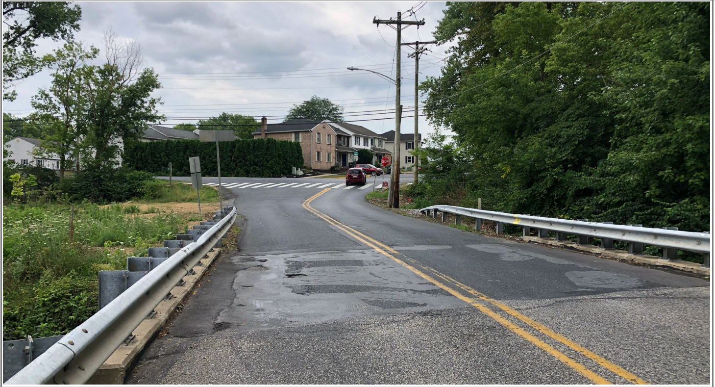
Photo 7 : View of Existing 22nd Street & Chestnut Street Intersection
