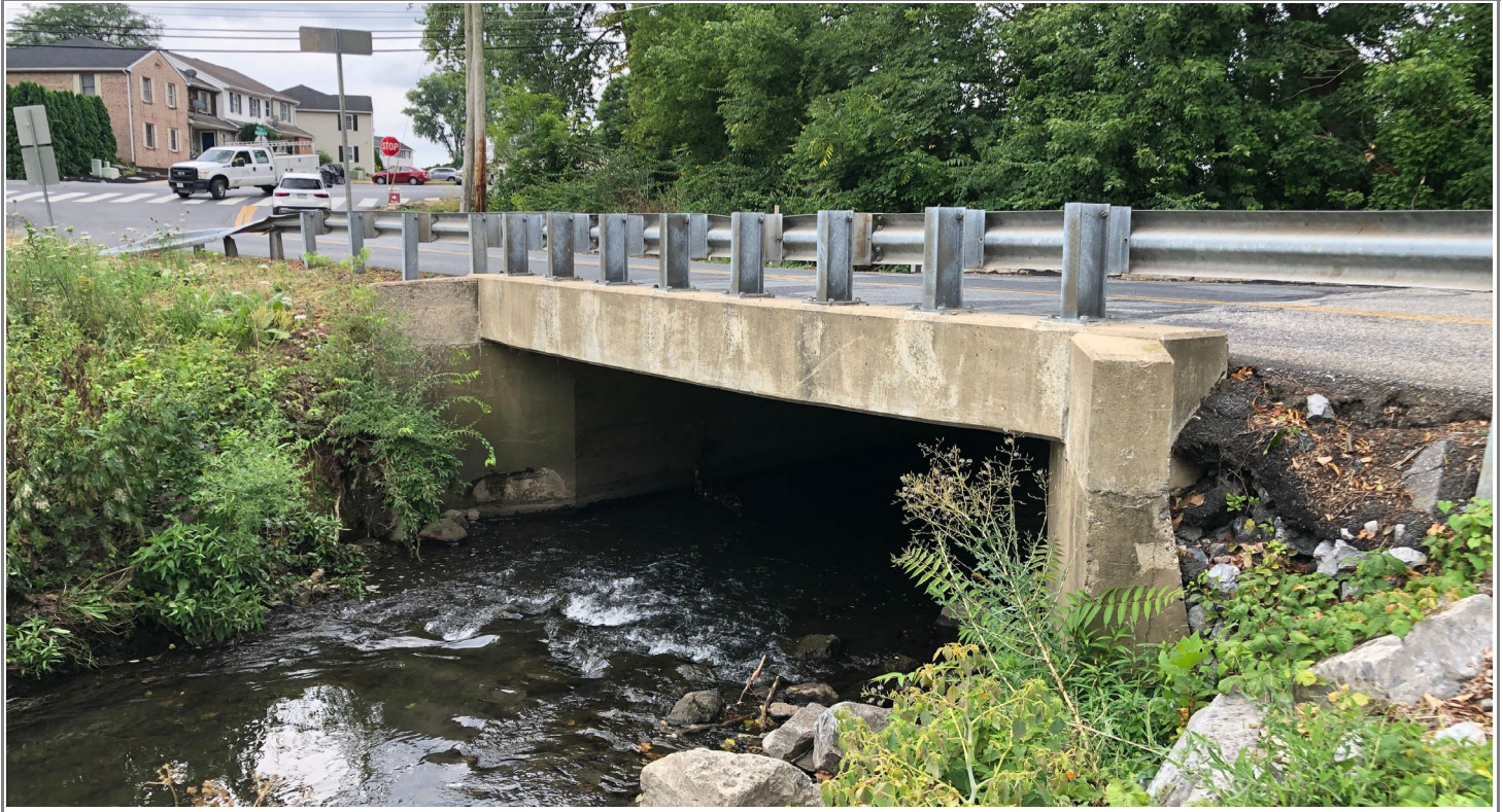
Photo 3 : View of Existing Bridge Over Quittapahilla Creek (Upstream Side)
