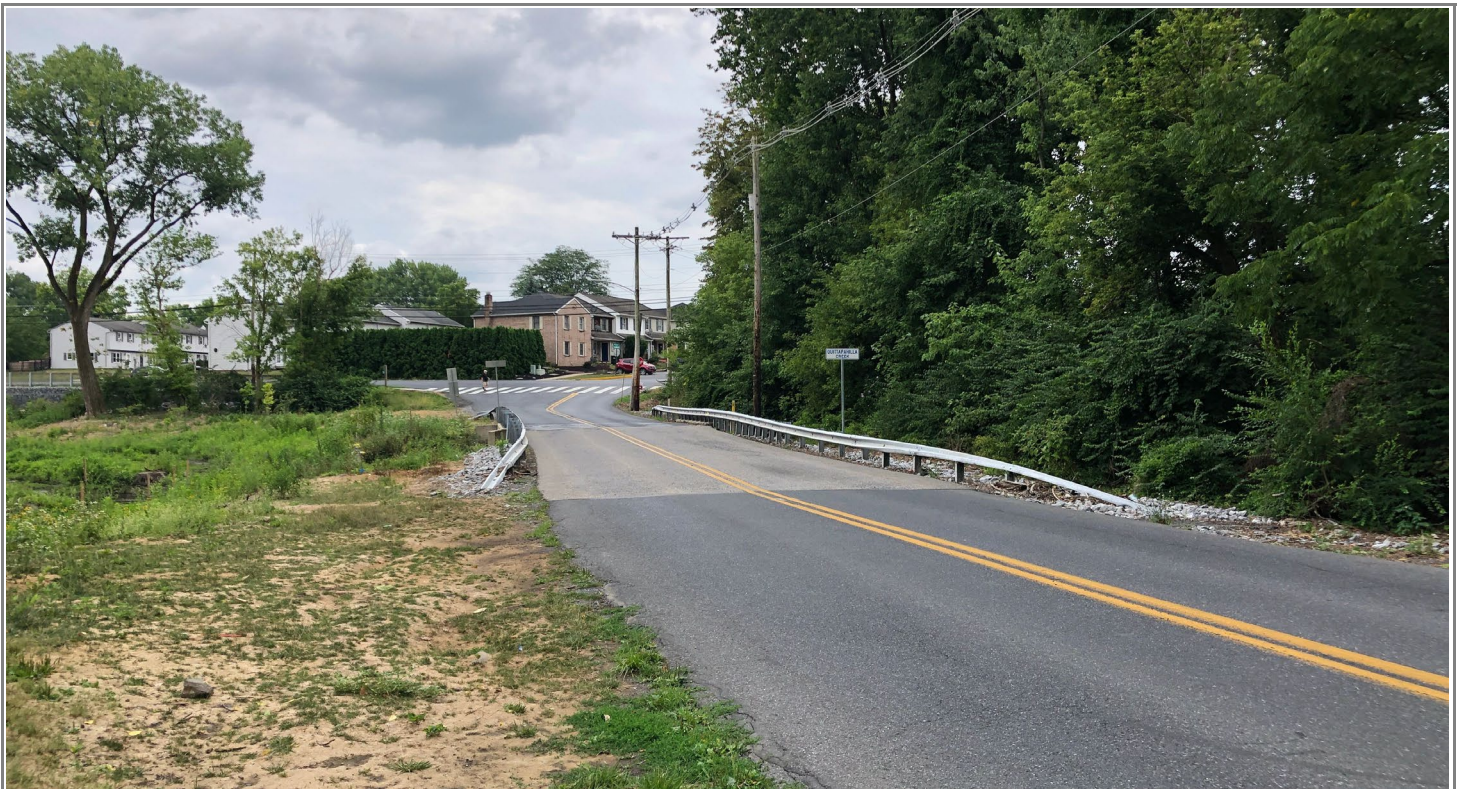
Photo 2 : View of Existing Bridge Over Quittapahilla Creek
