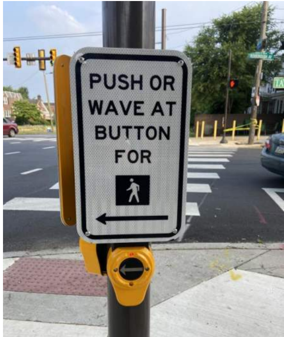
Accessible Pedestrian Signal (APS) Push Button (Broad, 9 th , 8 th Street) 无障碍行人信号 (APS) 按钮
