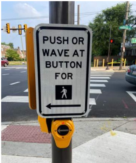
Accessible Pedestrian Signal (APS) Push Button (Broad, 9 th , 8 th Street)
