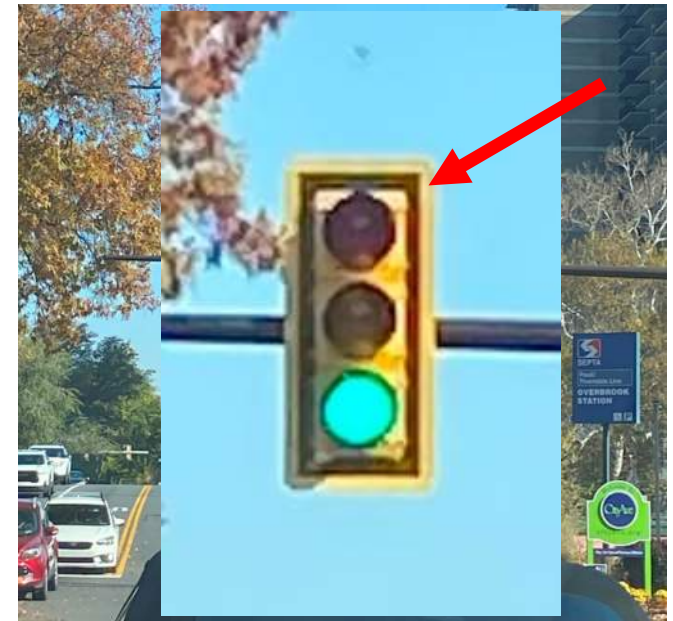
Retroreflective Backplates (all intersections)
