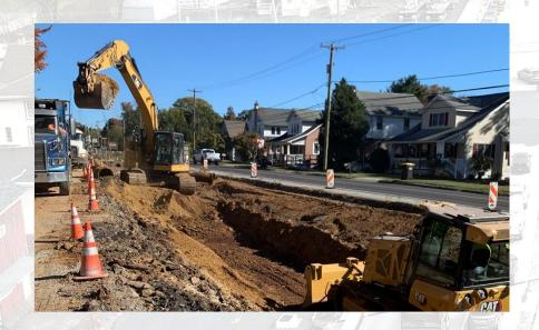
This fall, the contractor will continue with the excavation for the new noise wall, followed by the construction of the cast-in-place concrete foundation slab and stem wall. Following construction of the noise wall, the contractor will begin the installation of the new drainage on the SR202 side of the wall. The contractor will also begin the installation of the new sanitary sewer system between Germantown Pike and McDonalds.
