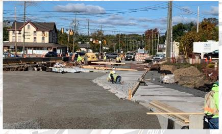
The contractor has also started the construction of the cast-in-place concrete sleeper slabs and approach slabs, after which, the remaining portion of the concrete roadway pavement will be constructed between the culvert and the SR202 intersection. Fine grading of the roadway subbase and placement of the new bituminous pavement, east of the culvert, will take place after the completion of the approach slabs.
