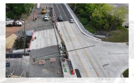
The contractor also placed concrete roadway pavement between the culvert and the Skippack Pike intersection.
