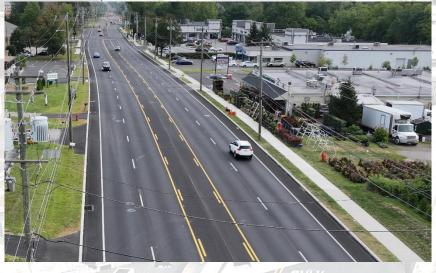
Profiling of the roadway and paving of the final wearing course, as well as placement of final pavement markings, remains to be completed between Skippack Pike and Jolly Road.
