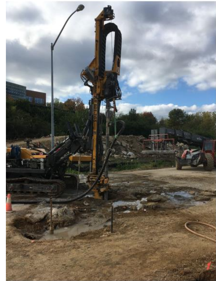
Typical grout hole drilling
