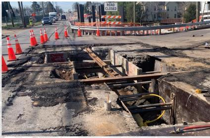
The contractor is also continuing with the installation of new water main and service laterals so the old main can be abandoned.
