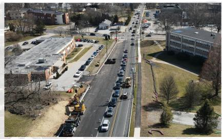
The contractor will also continue with roadway paving activities at the DeKalb Pike intersection, after the completion of sanitary sewer relocation work.
