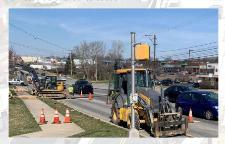
The contractor will also perform sanitary sewer relocation work in this area once the water and gas relocations are complete.
