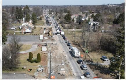
Once the sanitary sewer installation is complete, the contractor will resume the drainage installation and roadway paving activities between Johnson Highway and Hartranft Boulevard. The contractor will also continue with the construction of the precast concrete culvert top slab and backfilling, followed by remaining roadway paving north of Lawnton Road.
