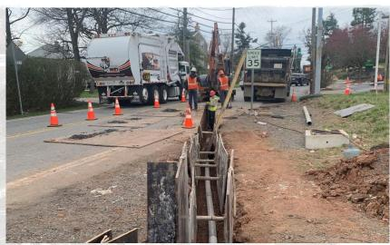
Following the relocation of the underground electric, PECO Gas will begin the relocation of the gas main and the transfer of services. Installation of the new sanitary sewer system will take place after the relocation of the gas main.
