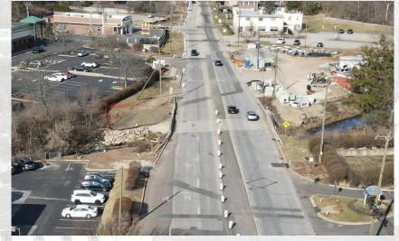
Once the water main relocations are complete and the old main can be abandoned and the contractor can begin the relocation of the new sanitary sewer system from Germantown Pike to McDonalds.
