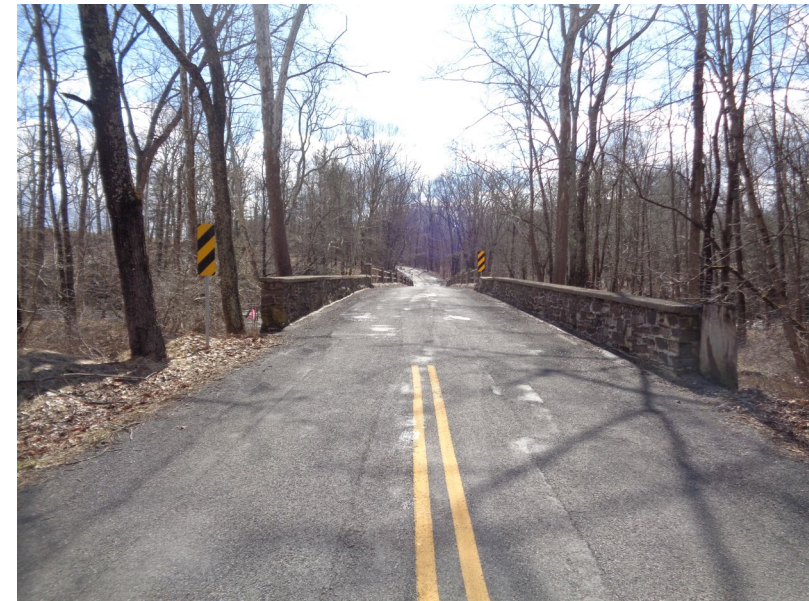
View of the north approach to the bridge, looking south.
