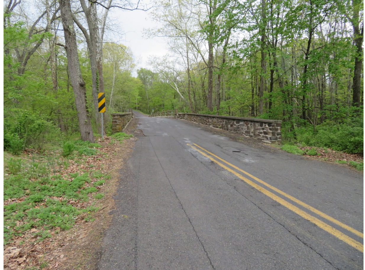
View of north approach to bridge, looking south
