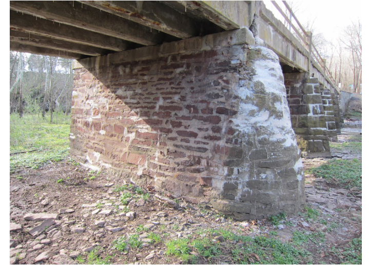
View of Pier 6 (Pier 1 is southernmost)
