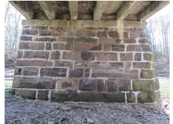
View of Pier 4 (Pier 1 is southernmost)
