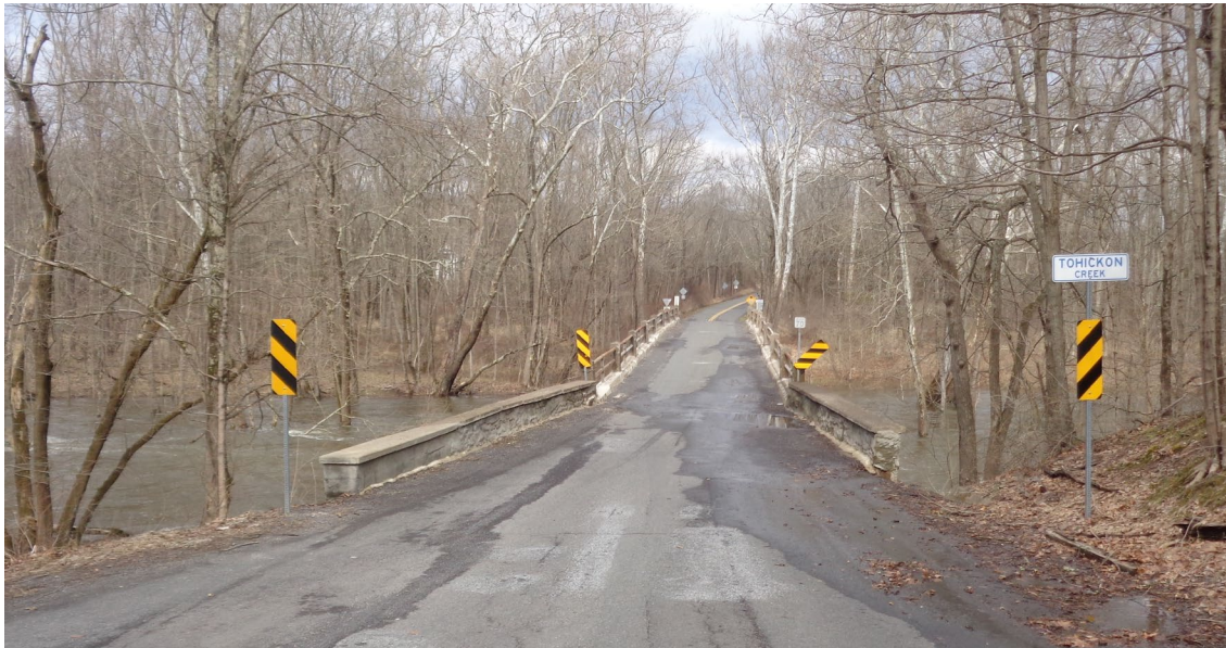
View of the south approach to the bridge, looking north.
