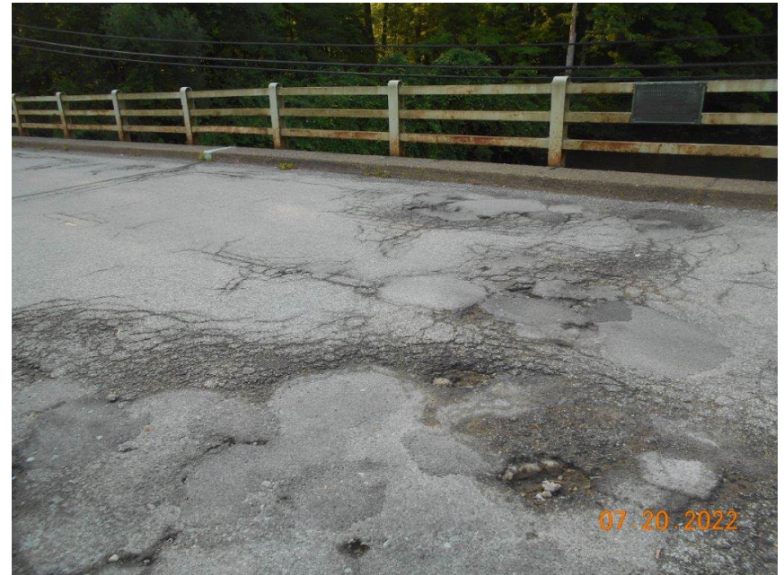
Existing Top of Deck
