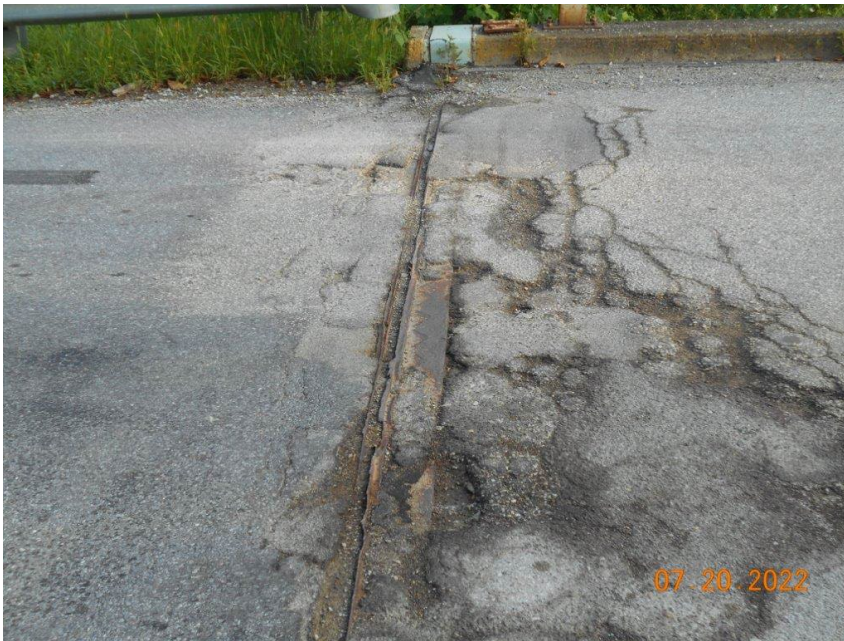
Existing Expansion Joint
