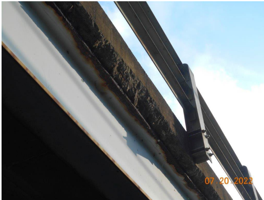
Existing Barrier Curb
