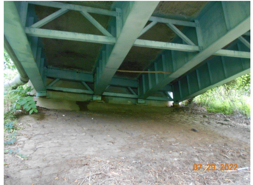
Existing Rocker Bearings
