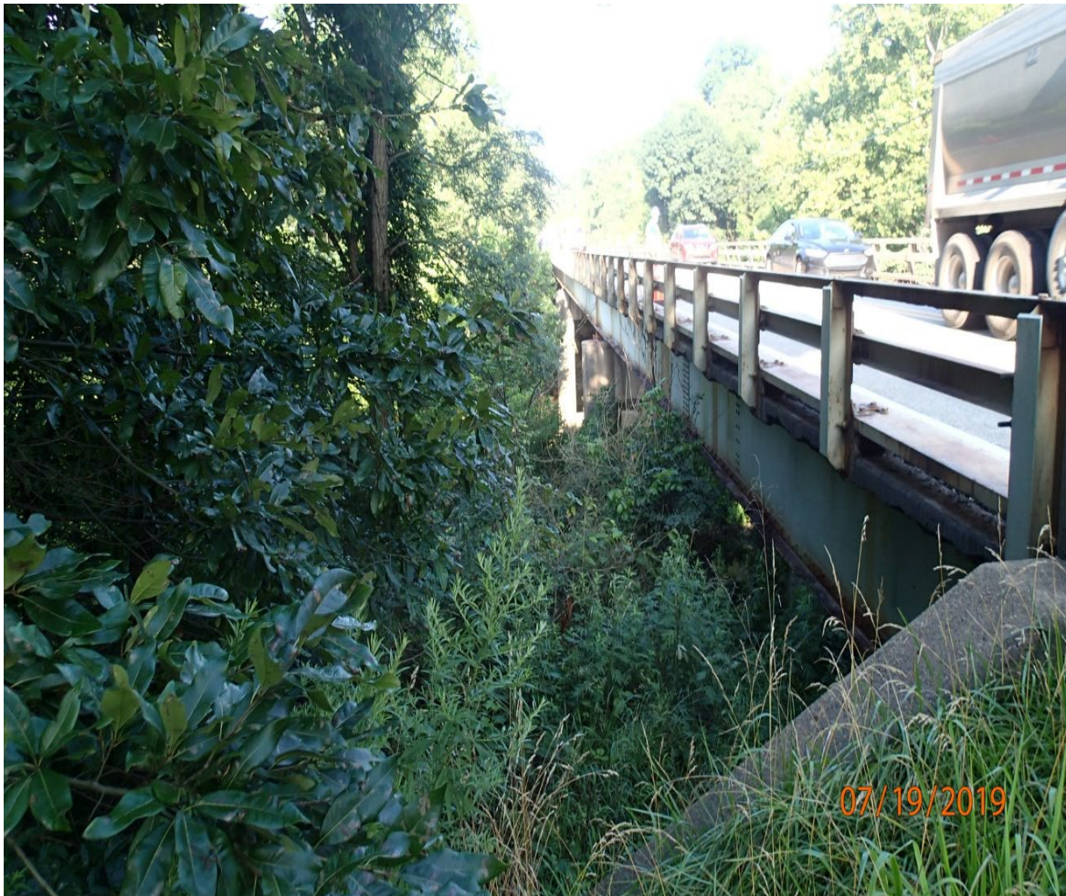
SR 1014 (Torrance Road) over MaGee Run Derry Township Built: 1952
