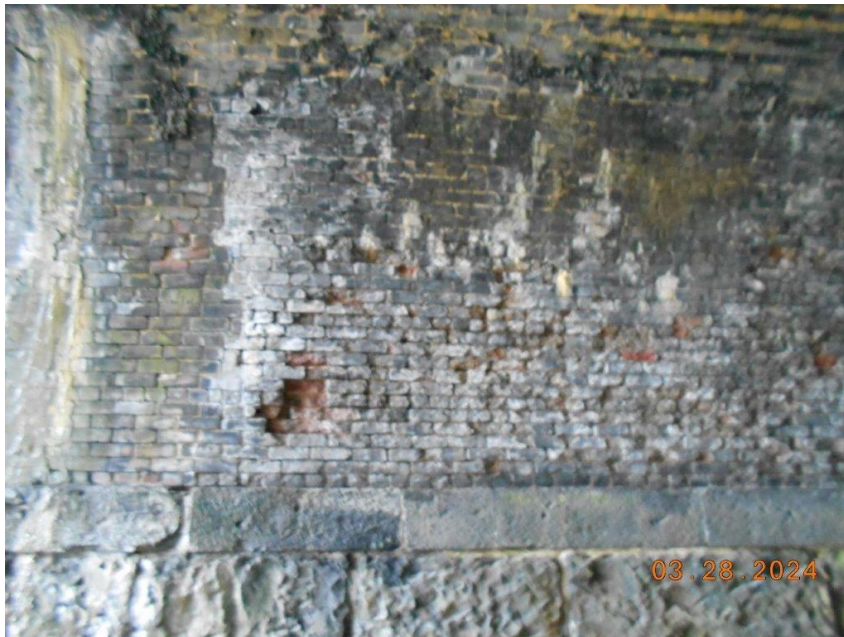
Deteriorated Brick
