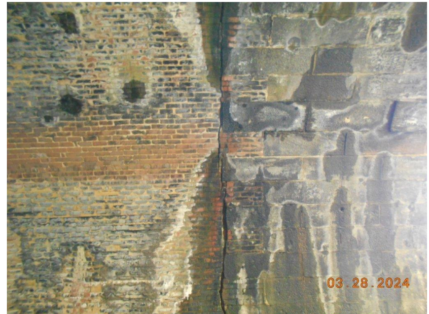
Ceiling Crack
