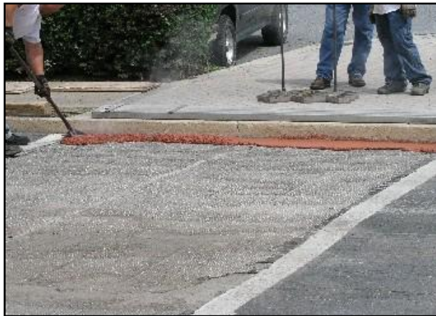
Photo 8, Molten asphalt is laid and spread
