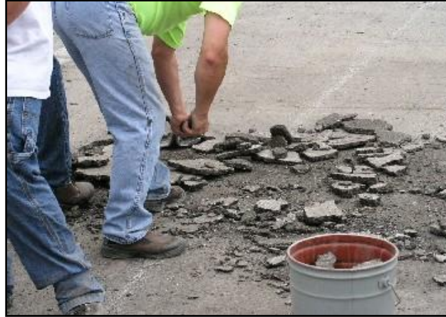
Photo 7, Removal of loose asphalt
