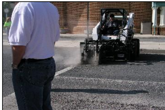
Photo 2, Milling existing pavement
