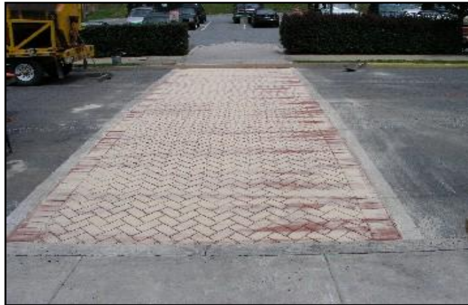
Photo 10, Completed overlay and imprinting.
