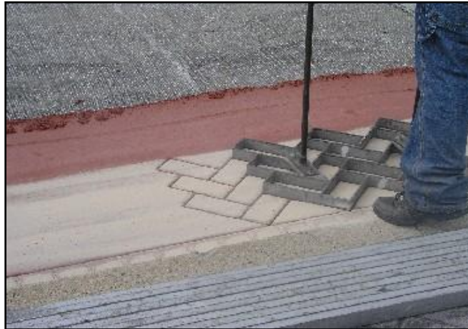
Photo 9, Brick design imprinting
