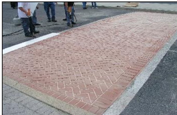
Photo 11, Application of thermo-plastic strips.
