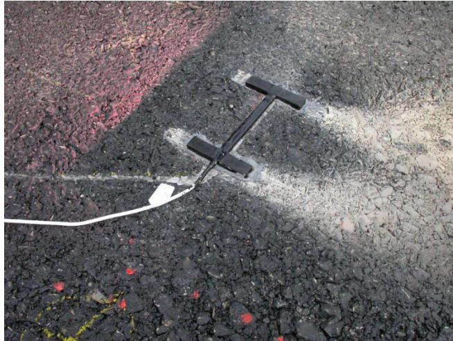
Figure 19. H-type Strain Gauge installed on the top of base course (Solaimanian et al., 2006).
