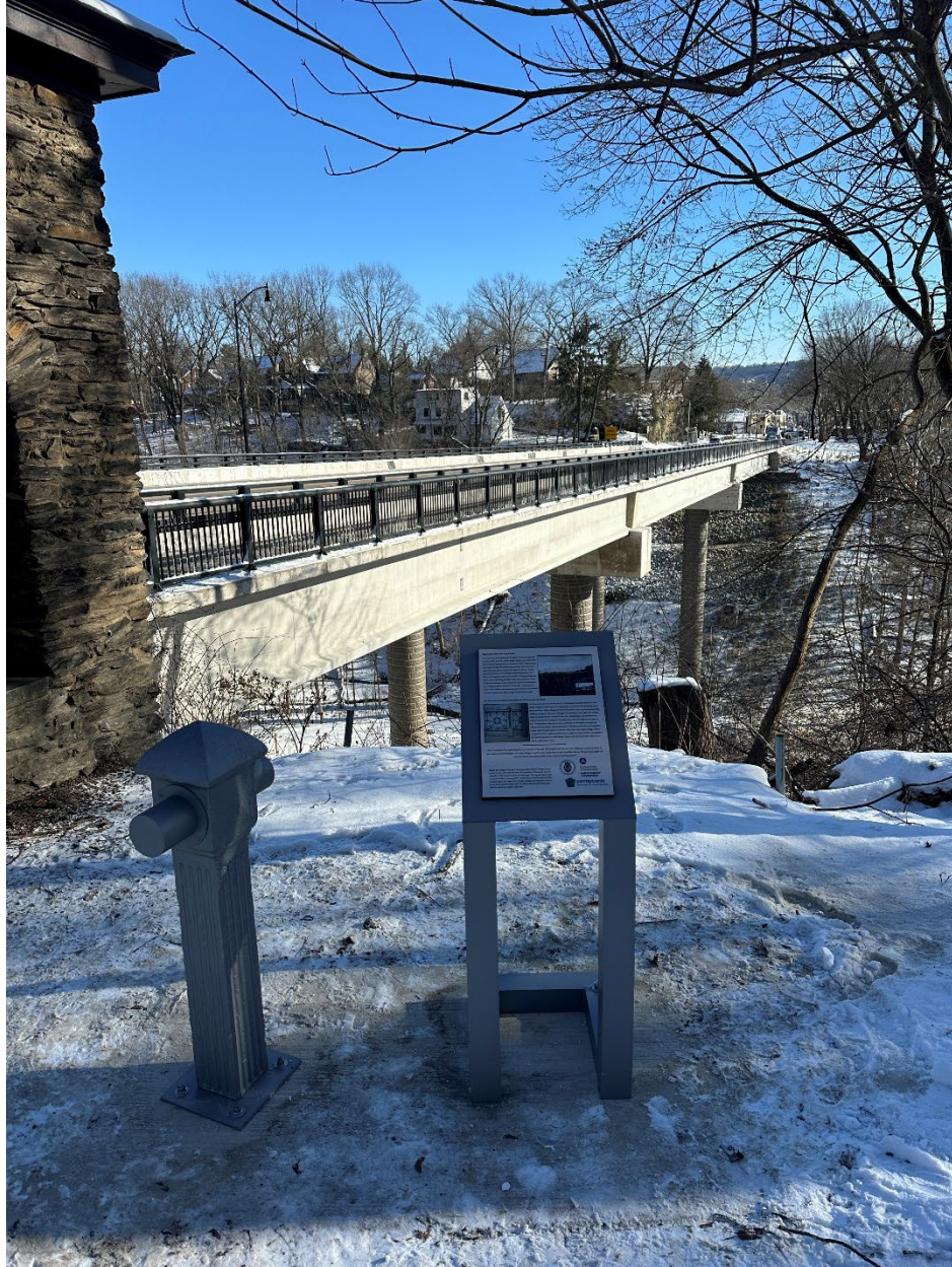
Fern Hollow Bridge in background with plaque and earlier bridge part in foreground.
