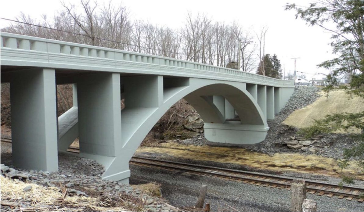
SR 4005 in Lackawanna County after Rehabilitation
