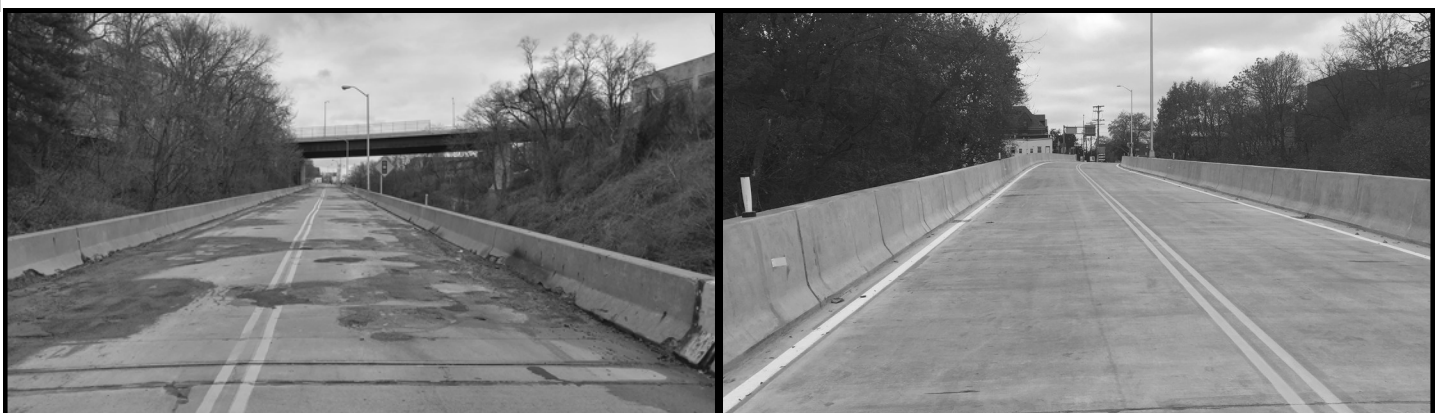
Neville Ramp Bridge before and after rehabilitation
