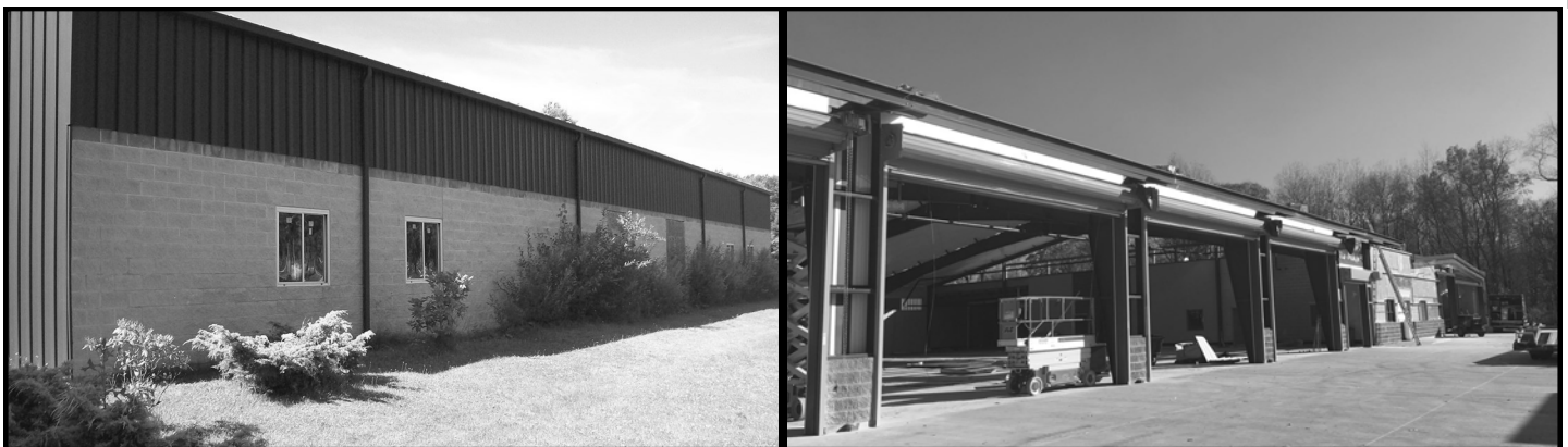
Crawford Light Maintenance and Storage Facility before and after rehabilitation
